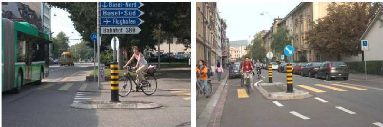
Figures 29 + 30: Secured oncoming bicycle traffic at intersections of one-way-streets (50 km/h), Weiherweg and Mülhauserstrasse, Basel
