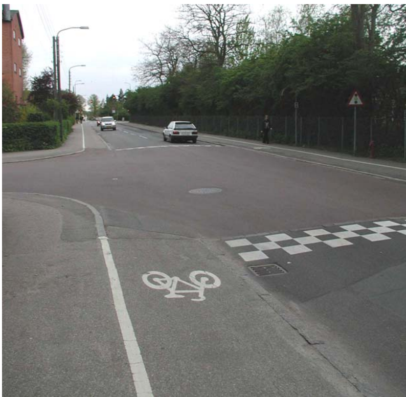
Raised intersection area with road humps established to slow down cars and thereby preventing accidents between cars and cyclists.
