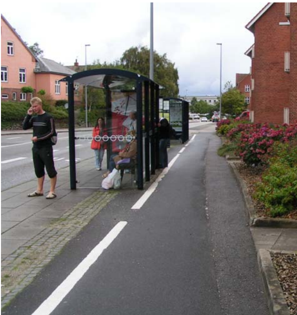
In order to reduce conflicts between bus passengers and cyclists, the cycle track has been positioned behind the bus stops and the footpath at some places in the city centre.
