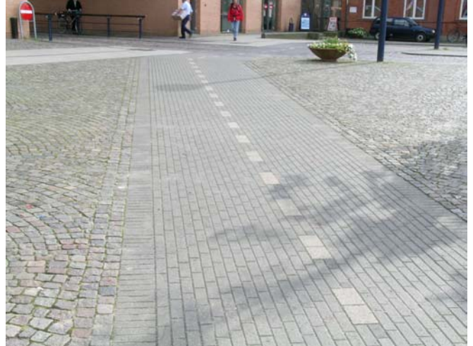
An untraditional solution using only paving differences has been used for a cycle track in the city centre.
